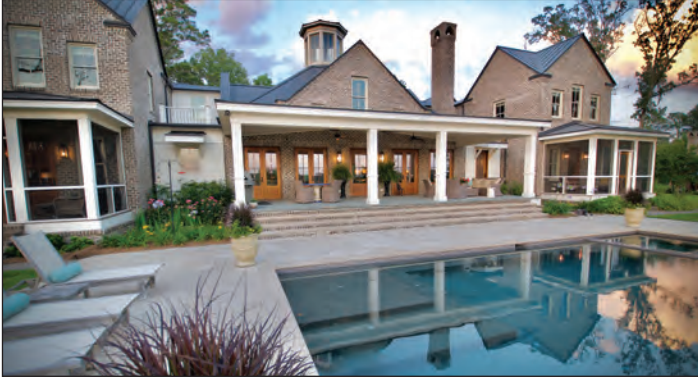
A large swimming pool and back patio overlook Rantowles Creek and provide sweeping sunset views of ancient rice fields.
